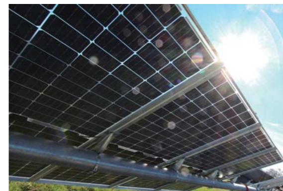
Bifacial module with transparent backsheet
